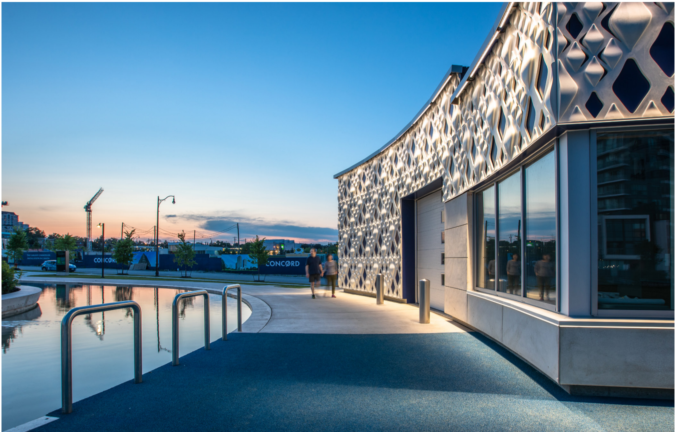
Figure 5. Droplet Pavilion - Curved Wall. Image courtesy of Concord Adex Inc.
